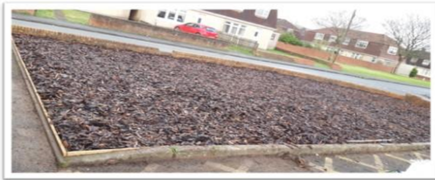
Upgraded area ready for phase 2
