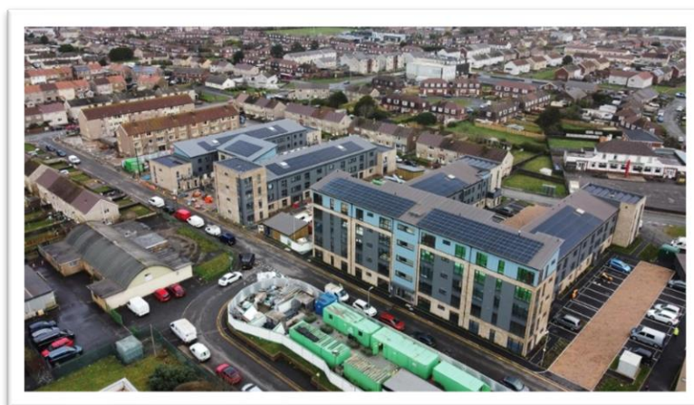
County Flats, Port Talbot, 2024
