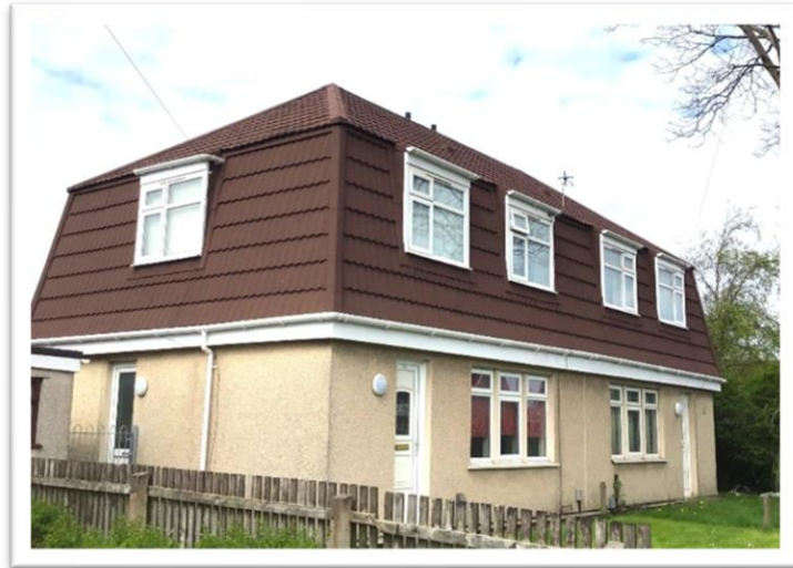
An upgraded mansard roof
