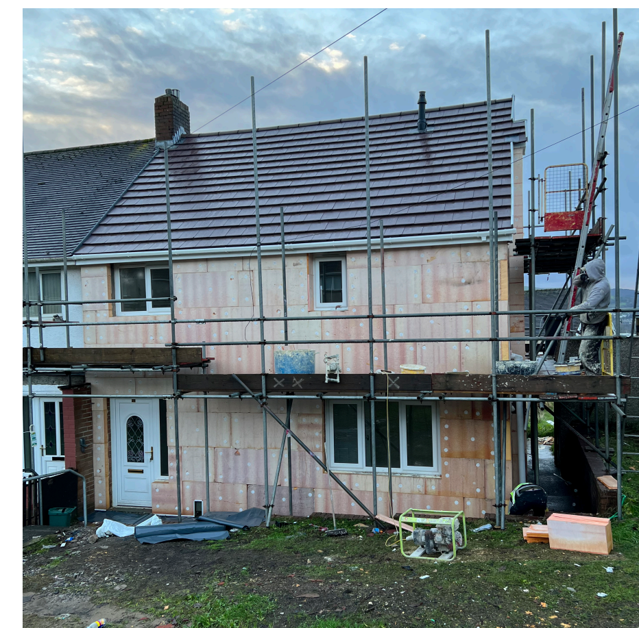
Progress at Caewern
