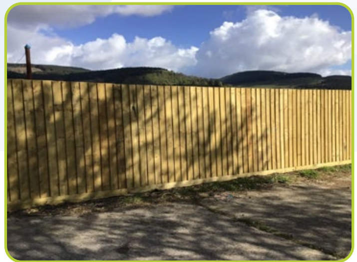
Tai Tarian completed Fencing
