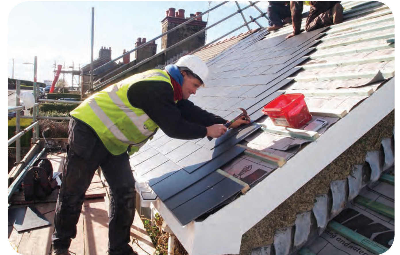
Roofing works to one of our properties
