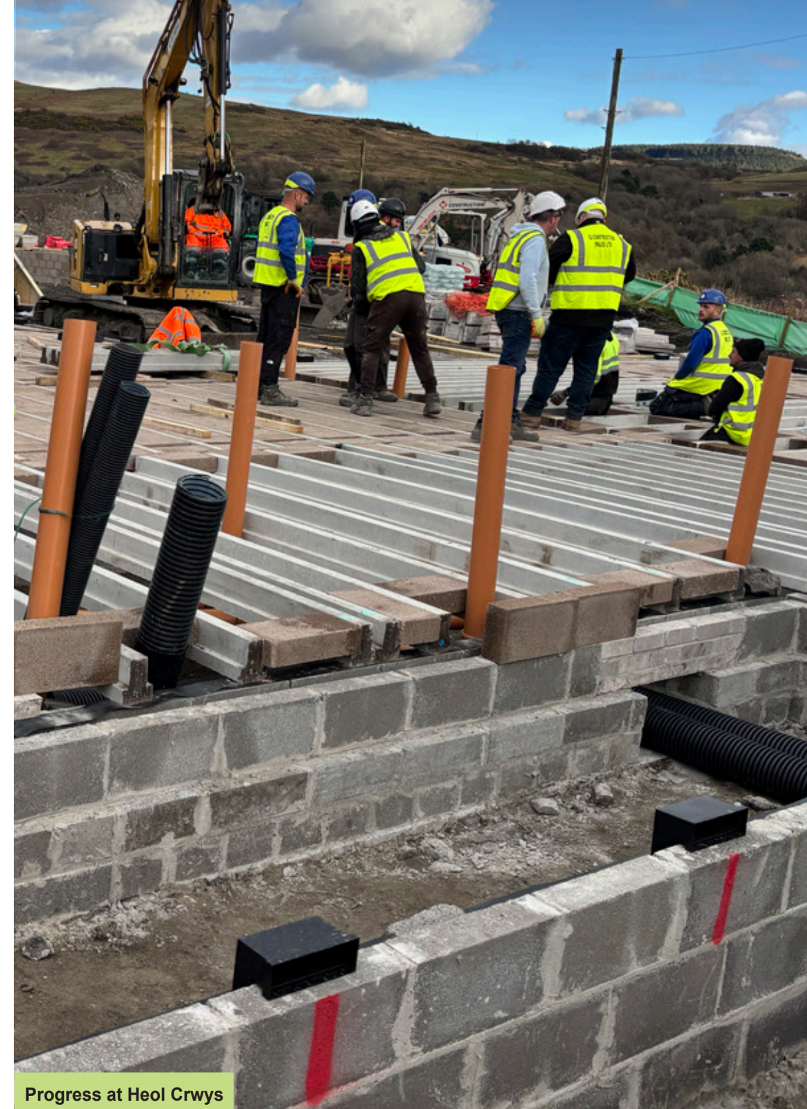
Progress at Heol Crwys
